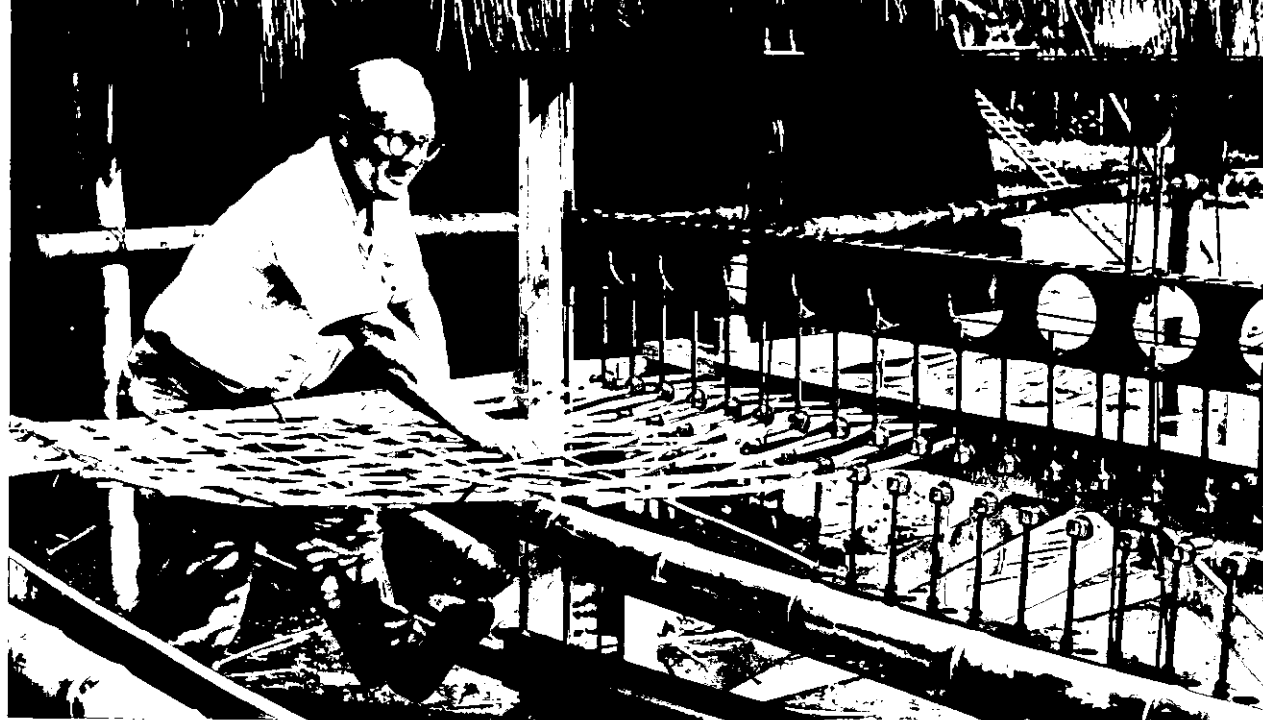
Bill Woudenberg at the loom he invented in Colombia. The loom weaves mats more than 6 feet wide and 14 feet long, each large enough to form the wall of a house.
