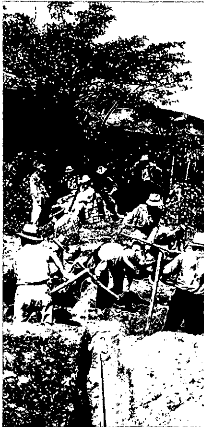
WORK PARTY digs a spillway hole, part of a Peace Corps-assisted aqueduct to bring water to village of El Chilcal from a mountainside source one kilometer away.
