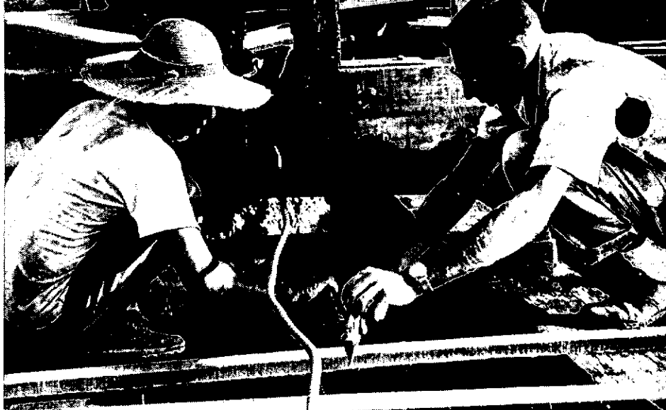
ALIGNMENT ASSIGNMENT finds Volunteer Bob Rourke using instrument to determine proper placement of piles for large aqueduct. The project is part of the Krian Irrigation Scheme, a program to increase the water supply to 60,000 acres of rice land in northwestern Malaya.
