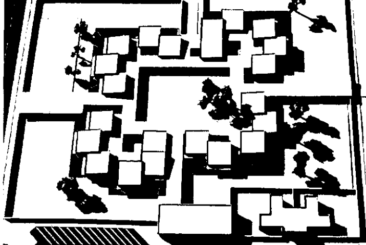
Grammar school for 800 students, designed by Jacques Ullman. Shed roofs are oriented to minimize strong south light.
