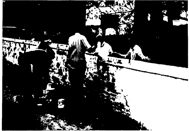
Staffers paint wall at HSC.
