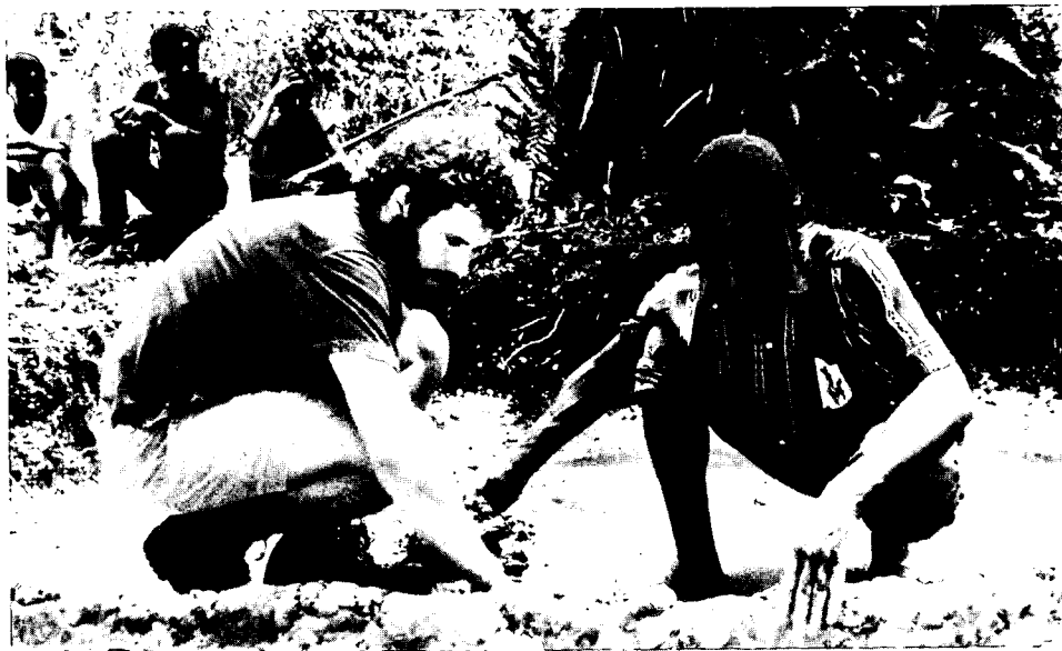
Glenn Lines, a water and sanitation Volunteer in the village of Kangu in Bas-Zaïre Region, here with his counterpart, is building a clay wall as the first step in capping a spring.
