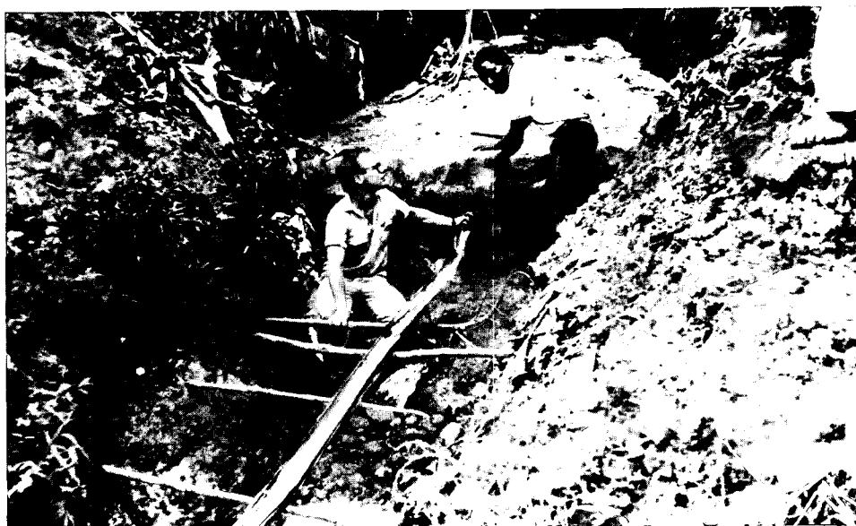
Water and sanitation PCV Tony Traverso and his counterpart Citoyen Buringo Byakunda organized the construction of two capped springs in the village of Kishondja in Nyabiondo. Here they examine a recently completed spring where the bamboo gutter, which protects the cement, is still in place. The spring will be covered with earth and vegetation as is the practice. Traverso studied at the University of Paris and holds degrees in philosophy and French from the University of Massachusetts, Boston
