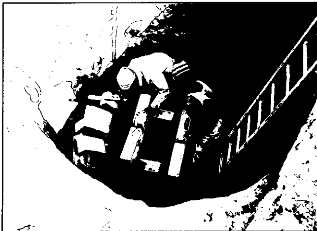
Two local masons constructing the soakaway pit for the new latrine project in Thies, Senegal.
