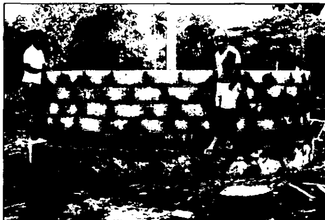
Constructing a water storage tank for the native species nursery near Puerto Ayola, Galapagos.
